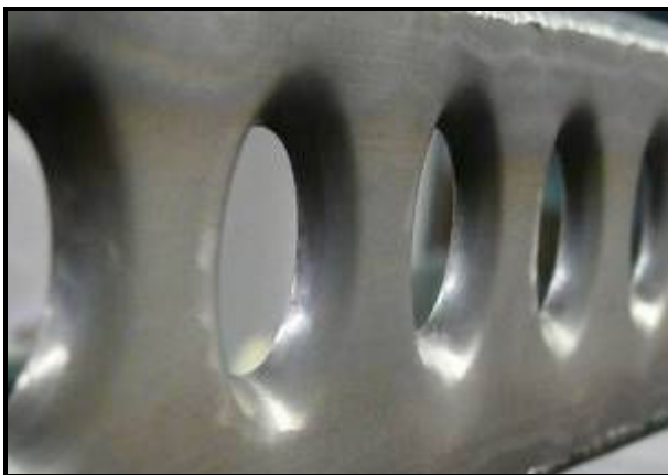
Figure 12: Flared Holes in Sheet Metal
