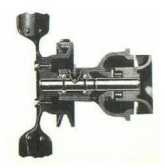
FIG. 15 —WATER PUMP ASSEMBLY
